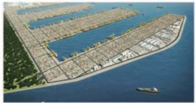
TUAS MEGA PORT Tuas South , Singapore
